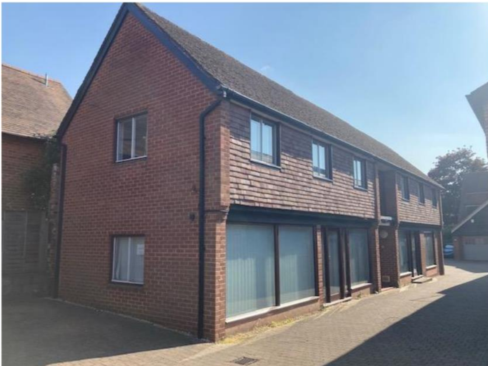
Photo of existing building
